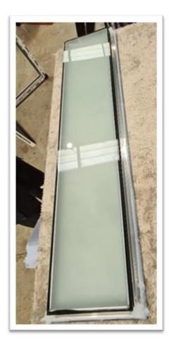
Once the silicone has been applied to the external cassette, Place the glass unit and external cassette into the external side of the aperture and firmly press against the cassette and slab to squeeze out any excess silicone.
