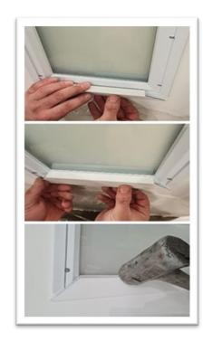
When re-fitting the cladding to the external cassette, ensure the first piece is spaced evenly within its keep
