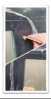
Clean the excess silicone from around the external cassette and glass unit using a rubber squeegee and wipes
