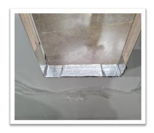
Remove the old layer of foil tape from the aperture and replace with a fresh piece spanning the width of the aperture.
