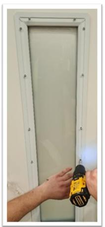
Line up the internal cassette centrally and within the aperture and screw into place using the provided screws.
