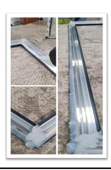
Apply a generous amount of silicone into the corners of the external cassette and along the inner channel of the external cassette.
