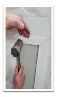
Tap the cladding into place with the use of a rubber mallet, taking care to only tap on the top side of the cladding.
