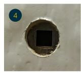
**4.** Once you have finished routing reinsert the locking mech into the door sash and check to see if the spindle aligns with the routed hole.
