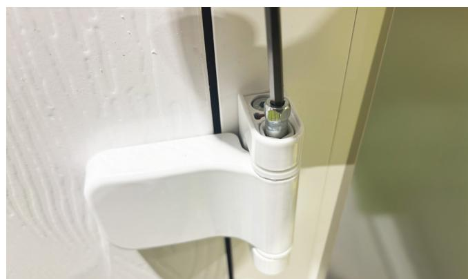
For compression adjustment, push the front hinge pin out and use a 4mm Allen key to adjust the compression. Once the adjustment is complete, push the hinge pin back in and replace the top and bottom hinge cover caps. Repeat this process for all hinges.
