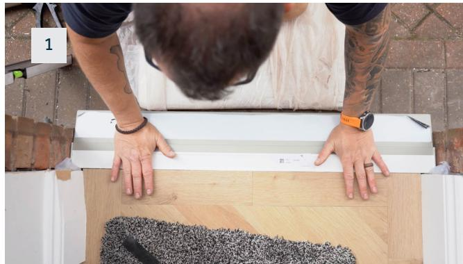
Place the PVCu cill onto the base, pressing down firmly to ensure it sits tightly against the packers and forms a strong, continuous seal with the silicone.
