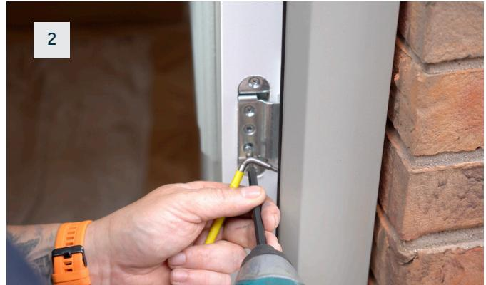
Loosen screws 1 & 2 by three turns. Tighten or loosen screw 3 with a 4mm Allen key to achieve the required adjustment.
