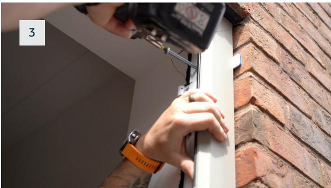
Pack between the frame and brickwork to ensure the frame is not distorted while fixing.
