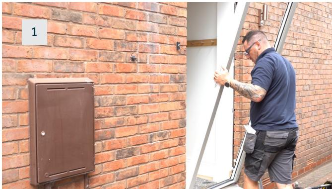
Lift the door onto the sill and temporarily secure it in position using timber wedges, packers, or an air bag. Ensure that the silicone seal between the bottom of the door and sill is unbroken.
