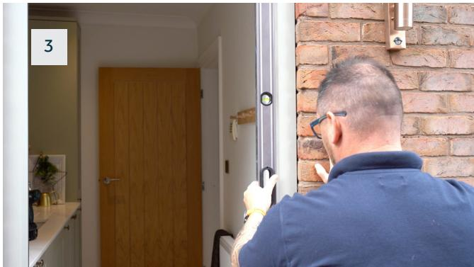
Once the hinge side is plumb, check that the frame is square by placing a 1.8m spirit level against the rebate on the hinge side frame.
