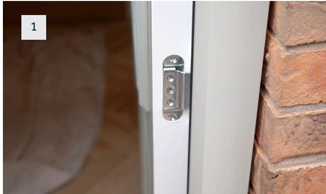
Due to the way SFS butt hinges are fitted into the slab, the lateral adjustment and margins are not set in the factory and must be set during installation.
