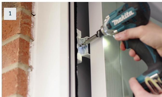
Remove the hinge cover retaining bolt using a No. 2 Phillips head driver. Then insert a 5mm flathead screwdriver under the cover cap and twist to pop the cover off.
