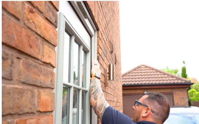
If you are using finishing trims, measure and cut the required lengths and secure to the installation using silicone.
