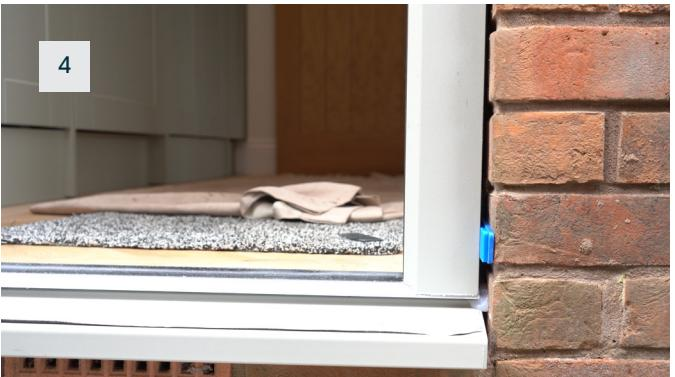
Pack all four corners between the frame and the brickwork to ensure the frame stays square and does not bend when fixing it to the brickwork.
