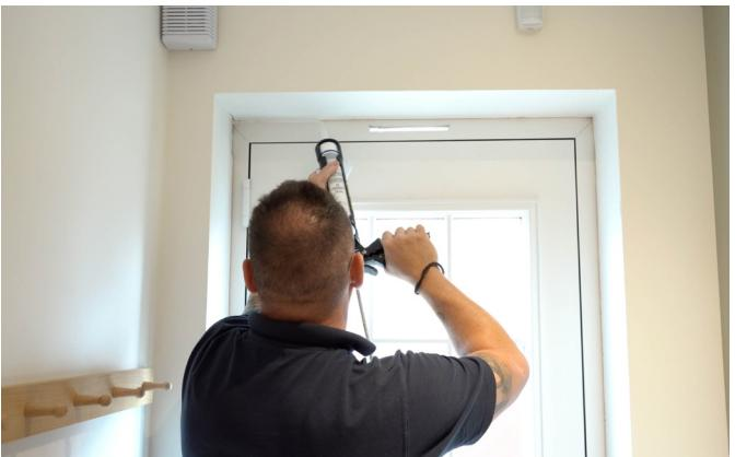
Replace the silicone in your gun with acrylic and use this to seal the gap between the door frame and the plaster line.
