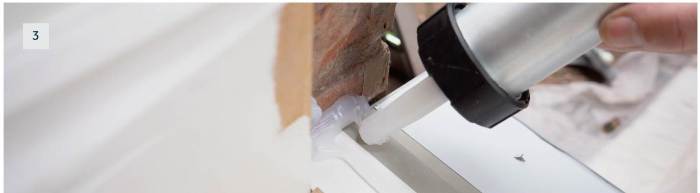
Apply a silicone seal approximately 10mm in diameter across the length of and ends of the PVCu cill to ensure a continuous seal once the door has been lifted into place.
