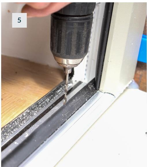
If you are installing onto a sill, drill three 4mm pilot holes through the threshold to fix the frame to the sill: one 70–90 mm from each corner and one in the centre. If the door you are installing has an aluminium threshold, take care not to drill through the thermal break.
