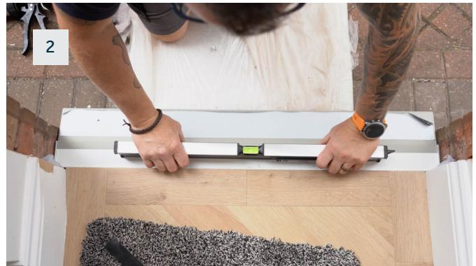
Check the level of the cill now that it has been installed and to ensure it remains 2mm higher on the hinge side.
