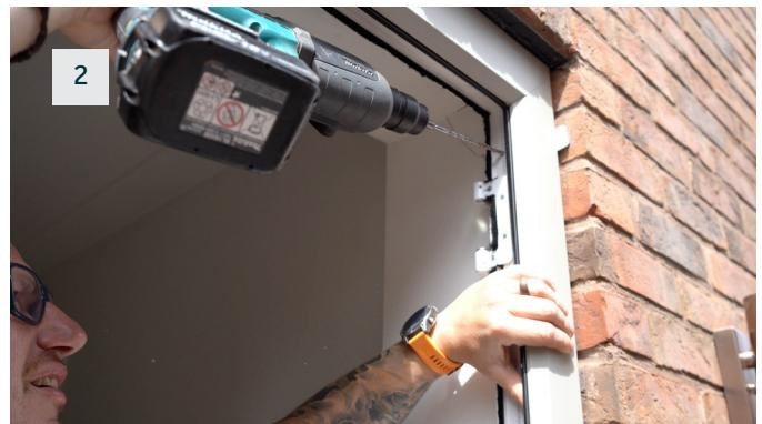
Use an SDS drill with a 6.5mm SDS masonry drill bit to drill into the pilot hole you have just created, ensuring you are penetrating at least 50mm into solid masonry, not into the mortar joint.
